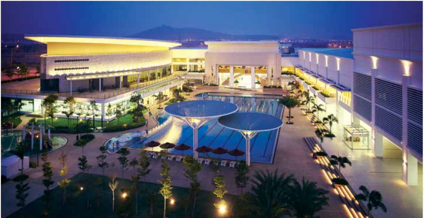
d'Tempat Country Club - A green building awarded Gold Standard certification (Provisional) by Green Building Index
