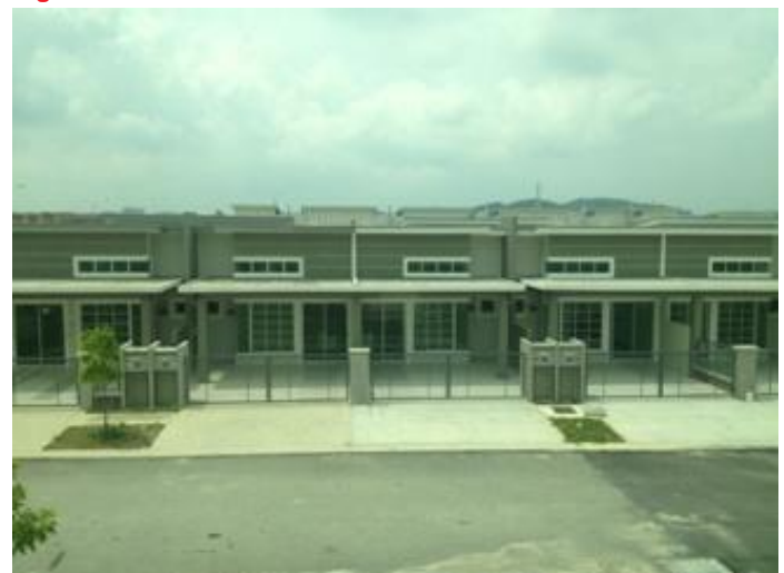
Figure 5: Link houses at BSS
