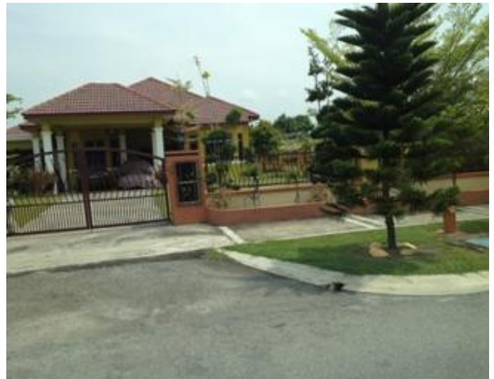
Figure 3: Bungalows built for Felda settlers
