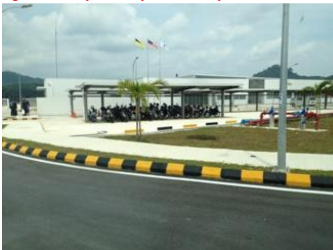
Figure 4: Factory at Sendayan Tech Valley
