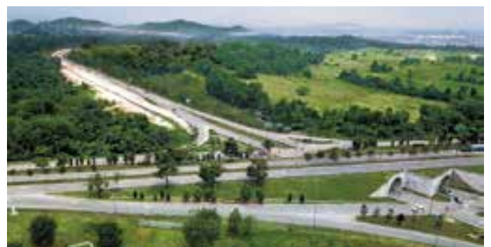
Persiaran Sendayan Mambau road upgrading works in progress
