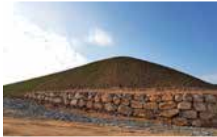
Boulders retention wall
