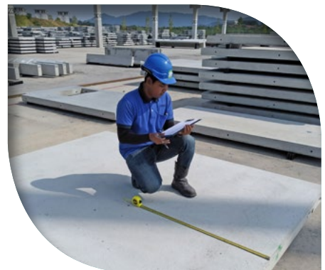
Industrialised Building System at work
