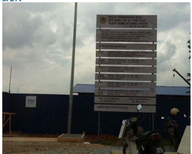
Figure 3: Messier-Bugatti-Dowty's plant under construction at STV
