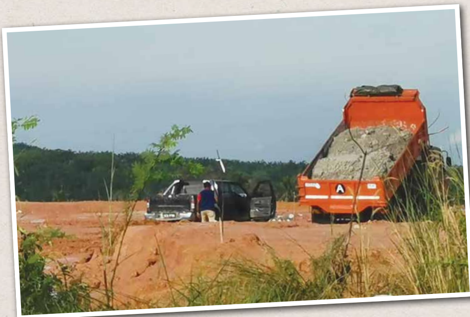
Re-using concrete waste for road underlay at construction sites.
